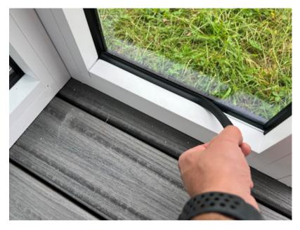
Remove the rail cover inserts by pressing the top of the cover inwards towards the glass or aluminum plate, the cover should easily snap free.
